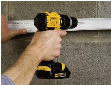
For engineering bricks, concrete and even steel reinforced concrete, the best solution when using the *Walldog®* is to make a 5mm pilot hole - again to 35mm depth.
