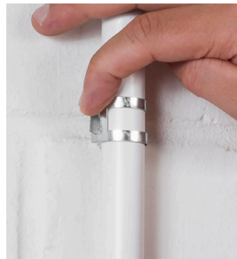
Secure conduit with locking tab
