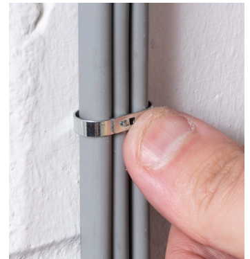
Push home to secure the Stag Clip and cable(s)
