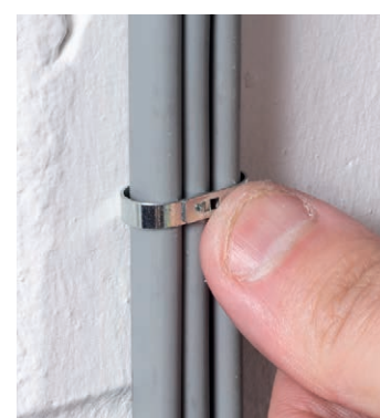
Push home to secure the Stag Clip and cable(s)
