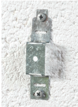
2x D-Fixings in Safe-D F-Clip 40
