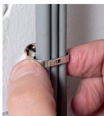
Insert cable(s) before squeezing the smooth head
