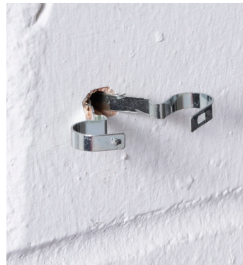
Rest Stag Clip in the pilot hole ready to accept cable(s)
