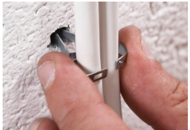
Push home to secure the Stag Clip and cable(s)
