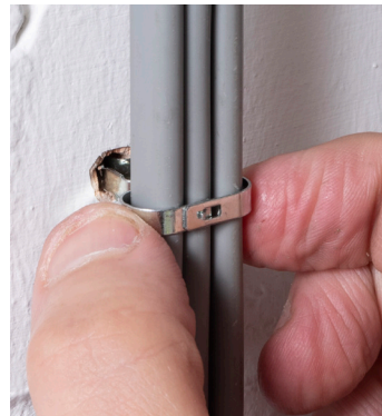
Insert cable(s) before squeezing the smooth head
