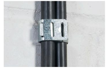
Safe-D F-Clip 30 & 40 are Fire-rated Flexible cable supports supplied in flat form, that can be quickly folded to secure cable installations.
