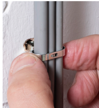
Insert cable(s) before squeezing the smooth head
