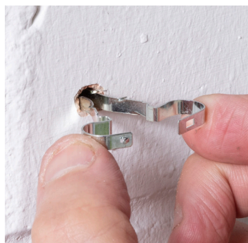
Drill pilot hole & select appropriate size of Stag Clip
