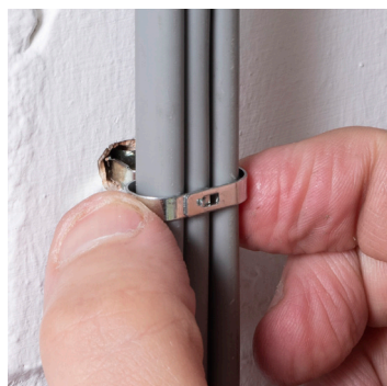
Insert cable(s) before squeezing the smooth head
