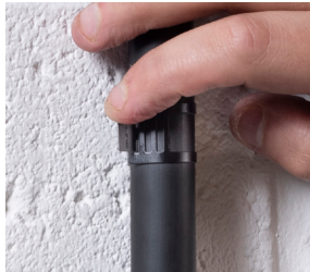
Secure cable with locking tab
